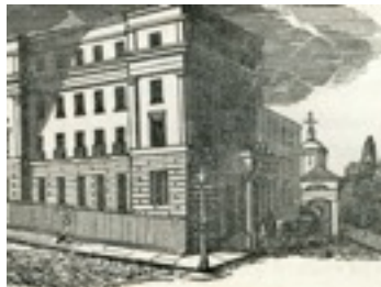
The weather vane can be seen on the right in this old engraving of the Regent Hotel
